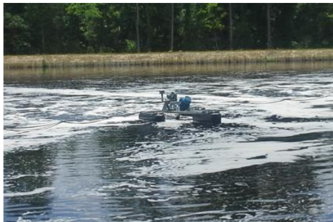
Example of Inefficient Surface Mount Aerator
